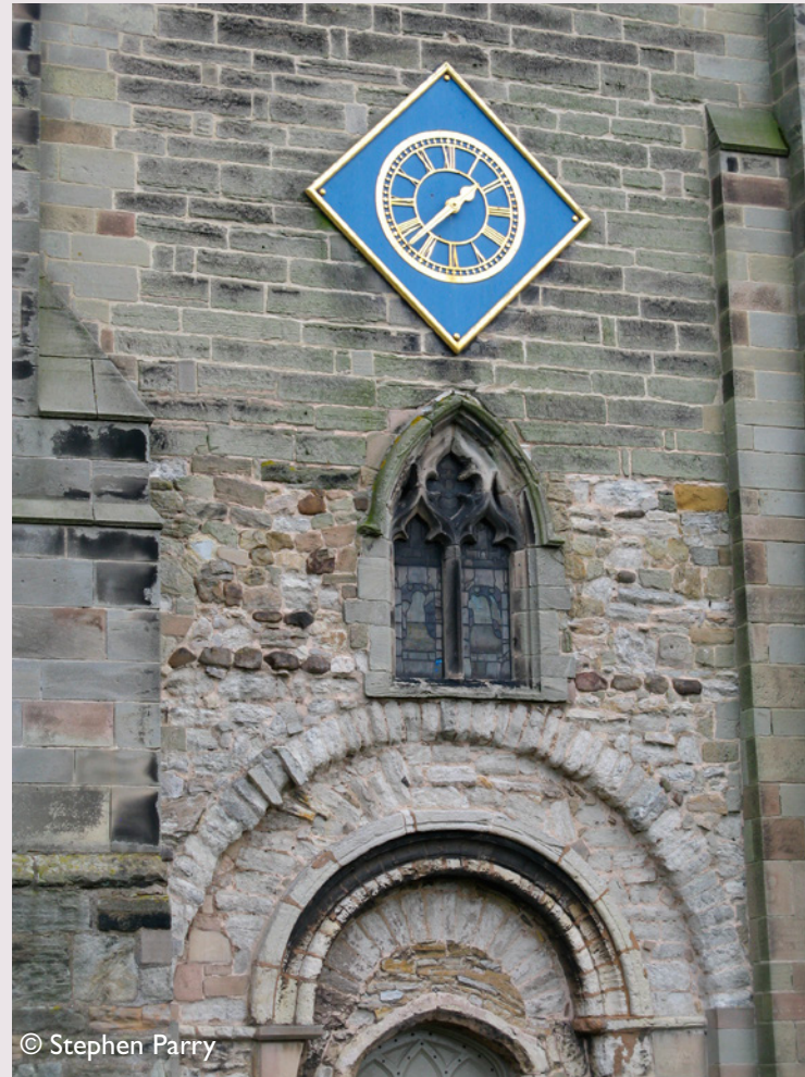
The Church of St. Mary the Virgin in Plumtree has Saxo-Norman origins and features locally gathered, reddened boulders of well-cemented quartzitic sandstone in both its tower and south aisle.
