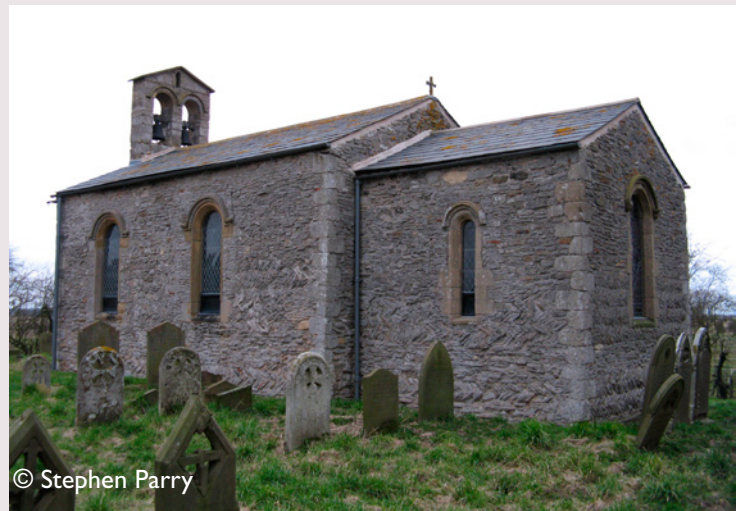
© Stephen Parry The Norman Church of St. Nicholas in Littleborough boasts extensive herringbone masonry of thinly bedded Skerry Sandstone.
