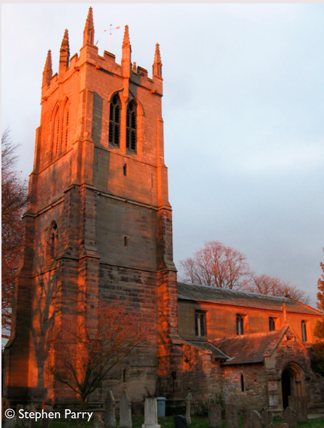
The massive C12 and C14, four-stage tower of the Church of Holy Trinity in Rolleston is constructed of pale Millstone Grit, which was quite clearly not quarried locally.
