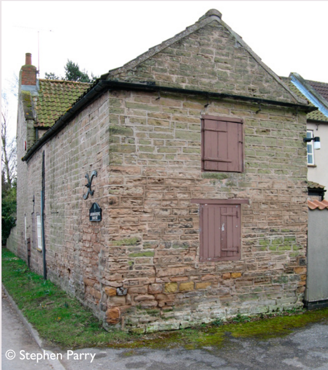
© Stephen Parry Asbourne House on Main Street, Edingley incorporates what may be a C17 coach house/stables, which is constructed of 'Waterstones Sandstone'.
