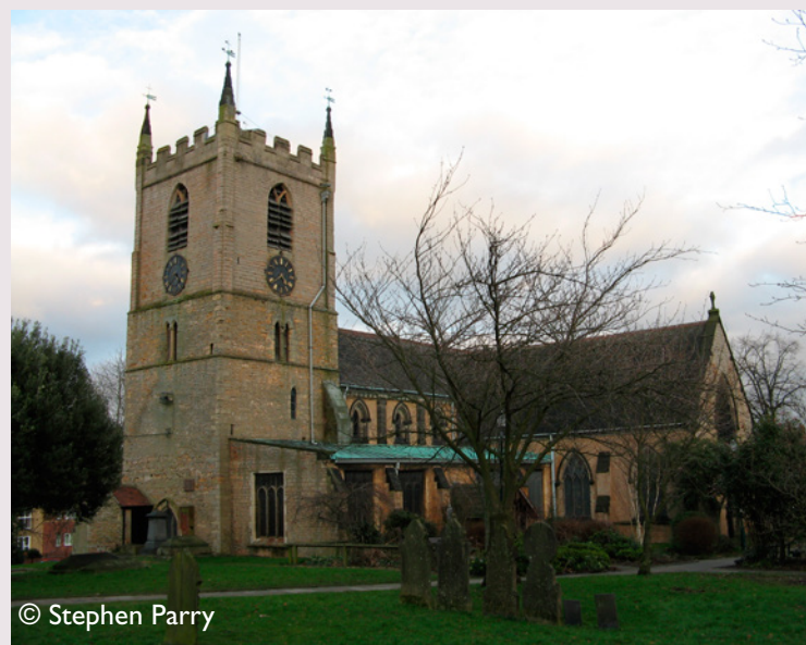
Locally quarried Linby Stone dominates the fabric of both the medieval and Victorian parts of the Church of St. Mary Magdalene in Hucknall.
