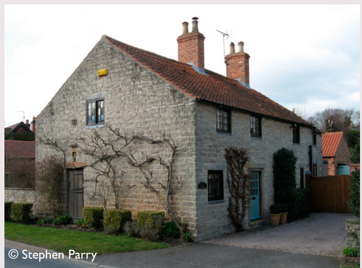
© Stephen Parry Use of 'thick-bedded' Skerry Sandstone was not restricted to churches, as is evidenced by various buildings, including Warrener's Cottage, in Thurgarton.
