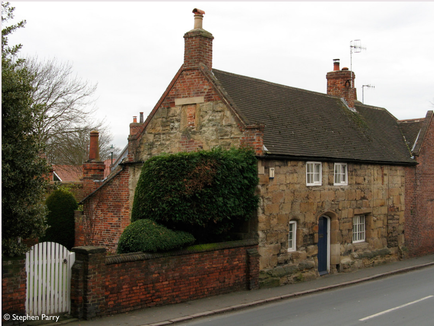
'The Chantry', a cottage located in Wollaton and dating to c.1500, is constructed of large squared blocks of Carboniferous Coal Measures Sandstone.
